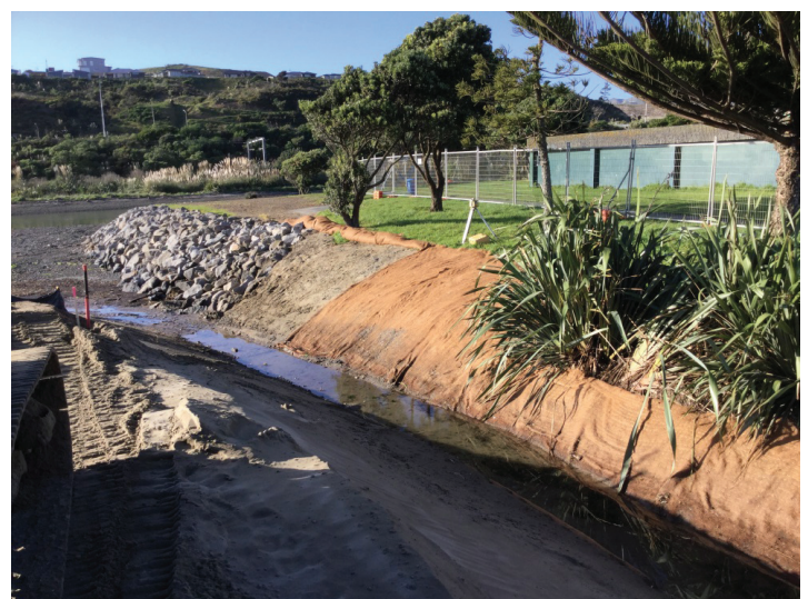
Inspection of coastal works in Porirua Harbour
