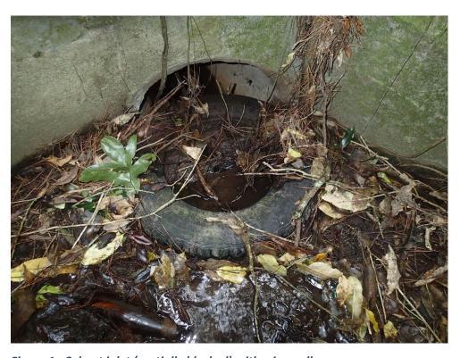
Figure 1. Culvert inlet (partially blocked) with wingwalls
