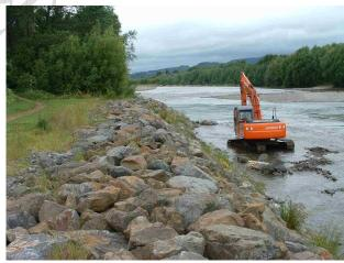
Maintenance – repairs to rock lining. Note platform formed in riverbed as machine is unable to work from the bank edge to rebuild this section of lining
