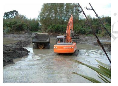
Silt excavation in Chrystalls Lagoon. Note use of self-draining weed bucket
