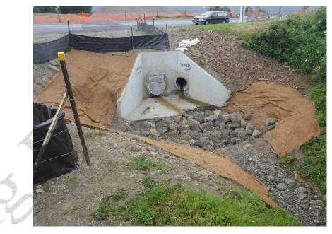
Silt fencing and ground stabilisation around newly installed wingwall
