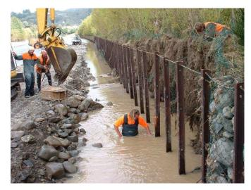
Formation of gabion structure; note separation of works from flowing channel and machine operating out of the water
