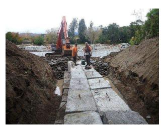
Foundation excavated and groyne core of concrete blocks placed out of flowing water
