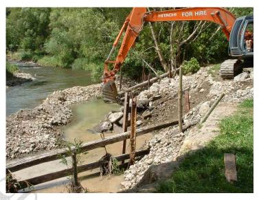
Repairs to timber permeable groynes on the Wainuiomata River. Note the separation of the work area from the active channel through the use of bunding
