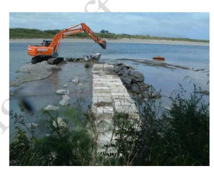
Groyne construction, showing use of bunding to protect works from flowing water and use of a formed working platform to elevate machinery out of flowing water
