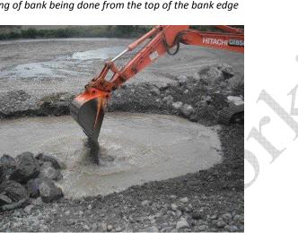
Excavating trench for foundation rock with machine located out of flowing water
