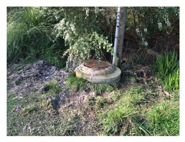
Figure 9. Un-constructed raw wastewater overflow discharging to the environment. Image courtesy of Steve Hutchinson, Wellington Water.
