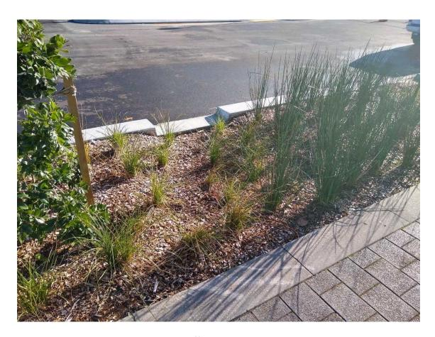
Figure 15. Raingarden treating road runoff.
