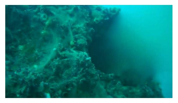
Figure 4. Moa point outfall discharging treated wastewater (image courtesy of Wellington Water, video available <a href="https://www.youtube.com/watch?v=9fKpdZVDIzc">https://www.youtube.com/watch?v=9fKpdZVDIzc</a>)
