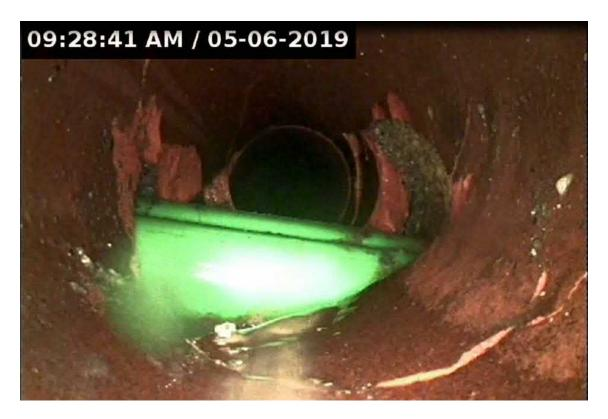
Figure 11. Strikethrough CCTV image within a wastewater pipe. Image courtesy of Steve Hutchinson, Wellington Water
