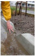
Scouring at raingarden inlets displaced mulch and soil (left). Stormwater inflow showing concentration of water to one side of the cut, but no scouring or leaf litter displacement (centre) and stormwater prevented from entering the raingarden due to overfilling with media/mulch (right). All photos in June/July 2008.
