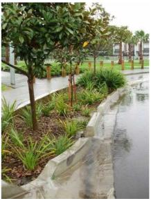
The combination of inlet placement and gutter design means most runoff bypassed this rain garden, so overloaded the next raingarden; blue marks indicate where new kerb cuts were to be made (left) 2008. Newly renovated raingarden with c. 150 mm of media removed except around retained trees and plantings, e.g. dense flax at the far end. New inlets improve flow from the street gutter (right) 2008.
