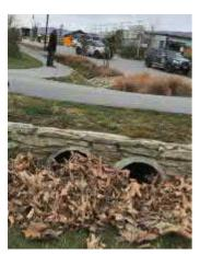
The most frequent maintenance activity is mowing grassed swales and removal of any debris in the swale systems (including slotted weir controls, pipes and cesspit inlets), approximately two-monthly, followed by trimming of hedges (although most hedges in
