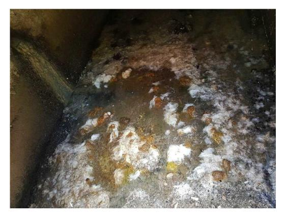
Figure 2. While shocking, this is the reality of an illegal cross connection in Te Aro (Wellington City) from a private residence, where their waste was being routed to a stormwater main. The next rainfall event would transport this to Wellington Harbour. Image courtesy of Steve Hutchinson (Wellington Water).
