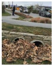
The most frequent maintenance activity is mowing grassed swales and removal of any debris in the swale systems (including slotted weir controls, pipes and cesspit inlets), approximately two-monthly, followed by trimming of hedges (although most hedges in
