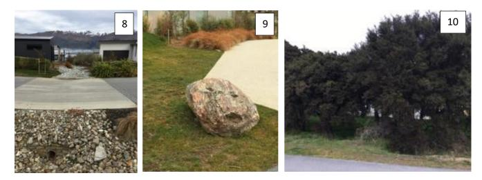
Photo 8: Fords for overland flow paths reduce need for pipes and are traffic calming features.
