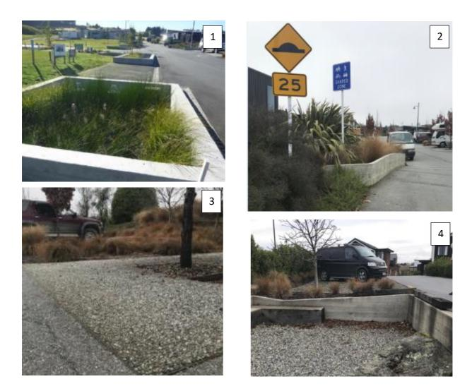
Photo 1: Stage 1 Rain gardens shortly after construction, before house construction showing raised edges.
