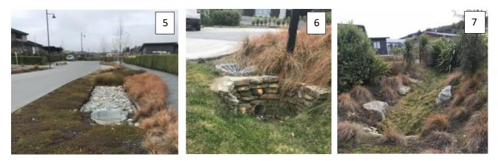
Photo 5: Raingarden with unplanted stone mulch and exposed overflow dome.
