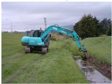
Figure 5-5: Vegetation and silt clearing from a drain beside the Hutt River
